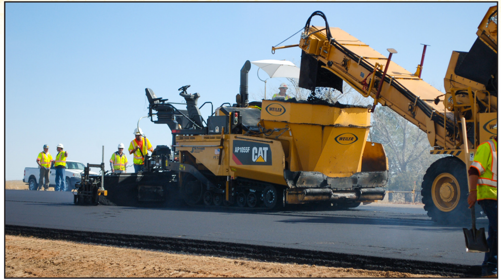
Paving Marksheffel Road
